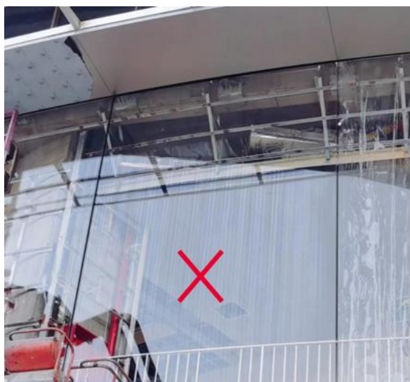
● 自然光下应力斑严重，目视清晰可见 Serious stress mark in natural light, clearly visible to the eye
