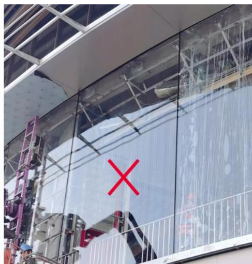
(偏振光下观察) 夹层边部效应—彩虹现象较重 (Observed under polarized light) Interlayer edge effect - heavy anisotropie
