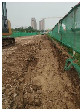
5. 坡顶排水沟开挖、砌筑、内外抹灰
