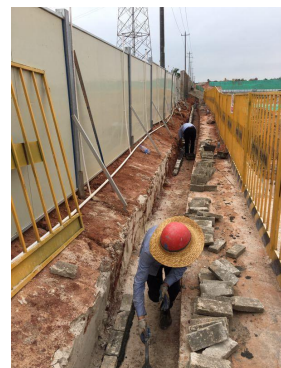
5. 坡顶排水沟开挖、砌筑、内外抹灰
