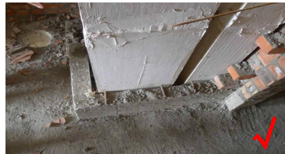
5. 烟道卸载应按每三层设置螺纹钢筋2条 \varphi \geq 10 ,一端架楼板,一端入墙不低于5cm.
