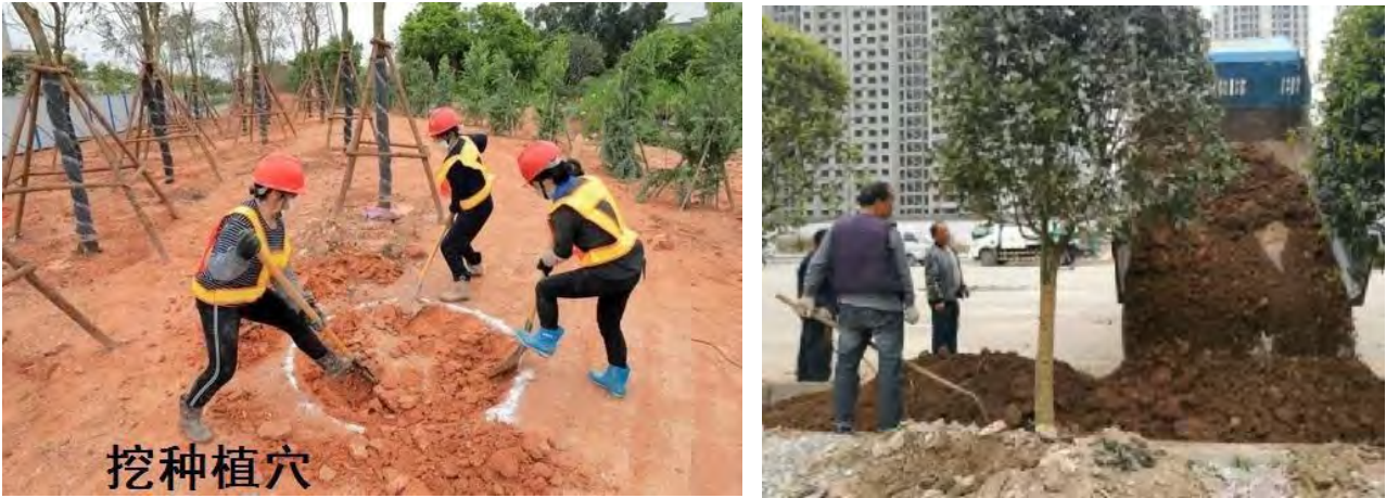
图5.5-6 挖种植穴客土回填
