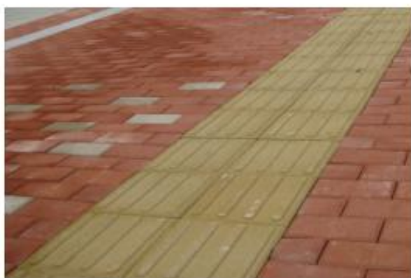
雨雪水通过砖体吸水，经过水孔直接渗透到地下。 Waters from raining and snowing will be copied by the tiles, then penetrate into the underground through water holes.
